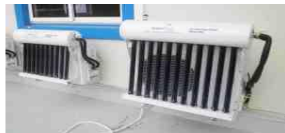
Fig. 5: Roof-top solar pv air conditioner
